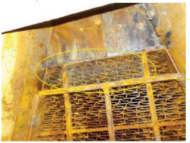
The "A" basket above this cold side basket is completely plugged and the sootblower cannot penetrate and prevent the accumulation of ash into the cold side which is fairly new.
