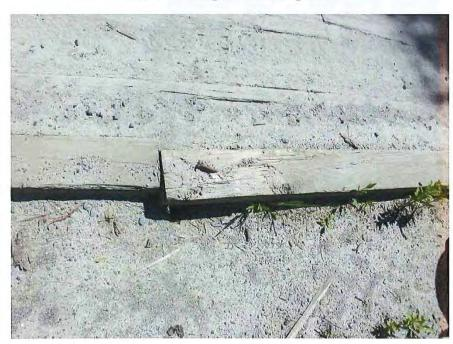
Photo 6 - Nails sticking out of wearing surface
