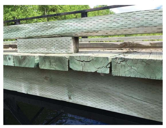
Photo 15 - TYPICAL CHECKING AT ENDS OF DECK SHEATHING
