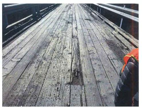
Photo 5 - TYPICAL DECK - WORN AND PUNKY IN SPOTS. LOOSE SPIKES.
