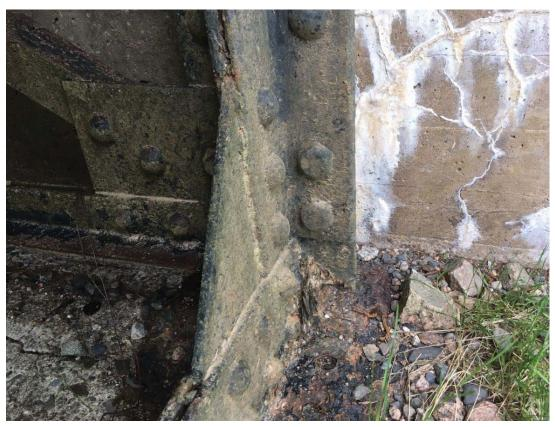
Photo 14 - SEVERE SECTION LOSS AT NW TRUSS BEARING VERTICAL
