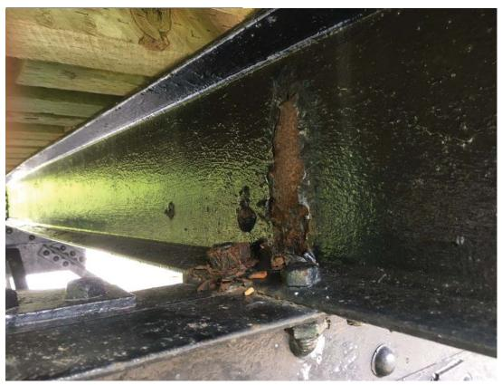
Photo 10 - TYP. CORROSION ON DECK BEAMS OPPOSITE BEARING STIFFENERS
