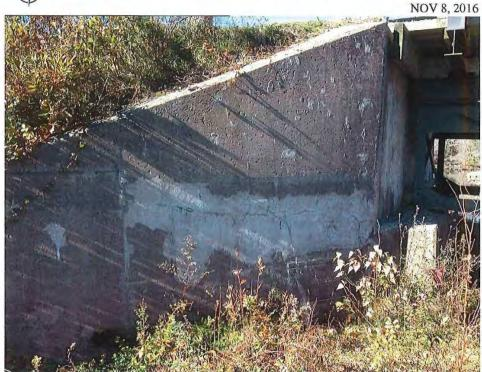
Photo 21 - SW WINGWALL REPAIRED
