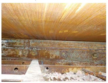
It must be noted that the hot baskets appear to be small in the compartments and this is demonstrated by the baskets all being stripped with perimeter sealing stripes to close off flow escape. This covers the stay plate welds and many welds could not be visually inspected.
