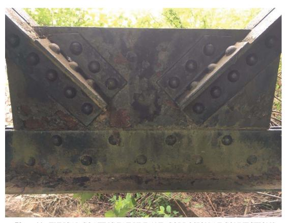
Photo 11 - TYPICAL COATING FAILURE AND CORROSION AT CONNECTIONS
