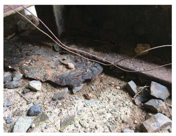
Photo 13 - SEVERE SECTION LOSS AT NW TRUSS BEARING PLATE
