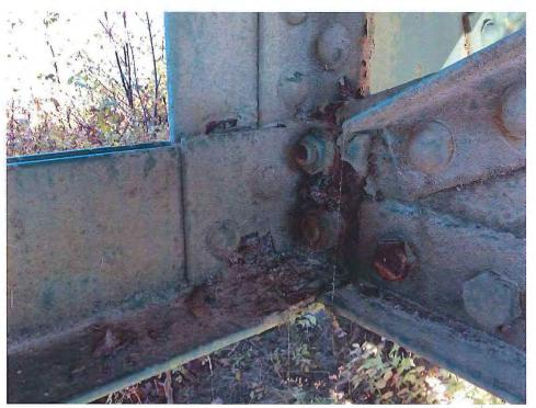
Photo 15 - CORROSION AT PANEL POINT, TYPICAL AT E END OF E SPAN
