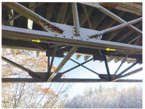
Photo 11 - PLATE WELDED ON BOTTOM CHORD IN SEVERAL LOCATIONS
