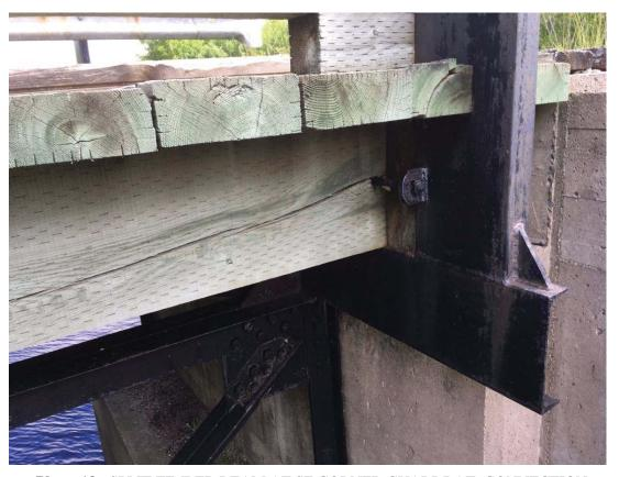
Photo 13 - SPLIT TIMBER BEAM AT SE CORNER GUARDRAIL CONNECTION
