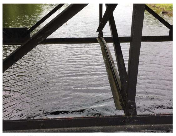
Photo 11 - DEFORMED BOTTOM CHORD OF WEST DIAPHRAGM BRACE
