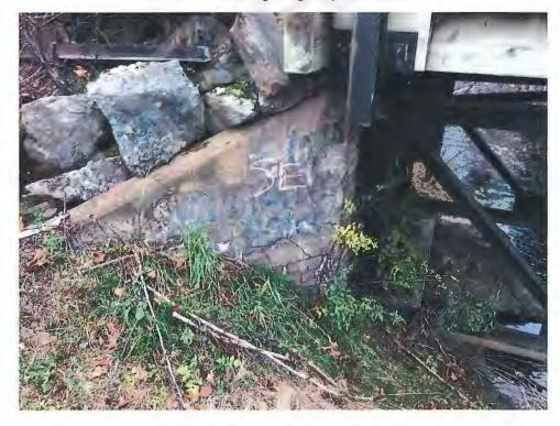
Photo No. 2 – Existing abutment wing wall.
