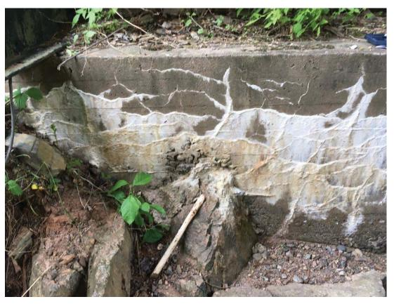
Photo 15 - E ABUTMENT CRACKING, EFFLORESCENCE, AND SEGREGATION
