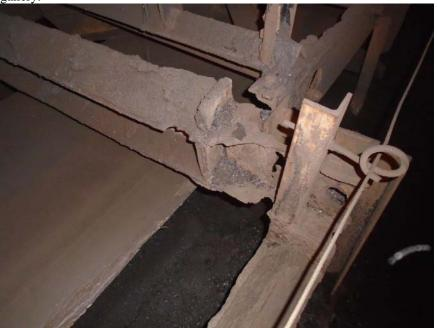
Corrosion around the flange of the coal chute where coal flows onto the E belt which takes the coal into the plant.
