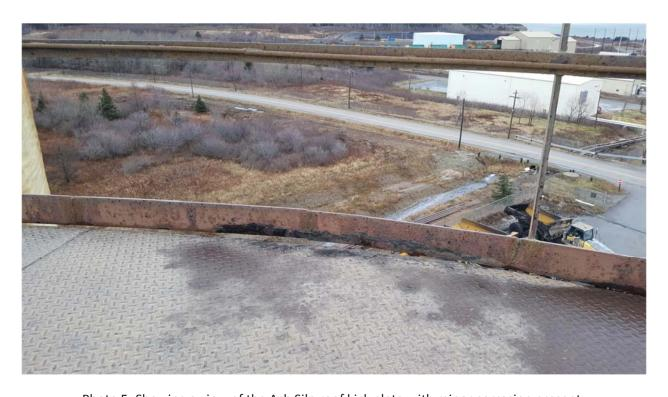
Photo 5: Showing a view of the Ash Silo roof kick plate with minor corrosion present.
