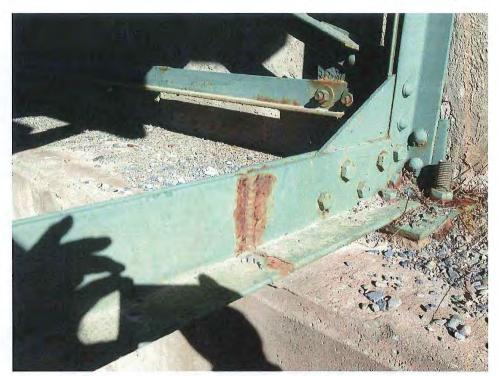
Photo 9 - PAST REPAIR TO BOT CHORD, SE BEARING ON E SPAN
