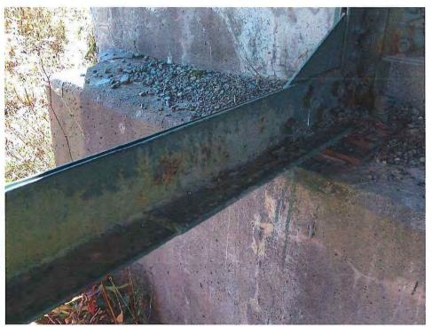
Photo 20 - PAST REPAIR TO SW BOT CHORD AT BEARING
