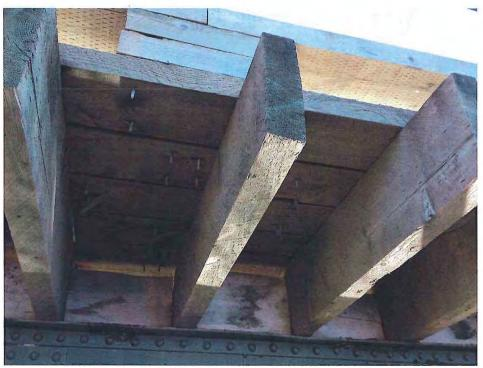
Photo 12 - TYPICAL UNDERSIDE OF DECK/STRINGERS
