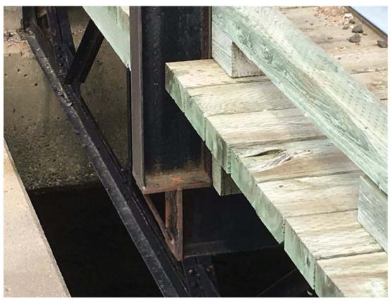
Photo 14 - WEAK STIFFENER DETAIL AT GUARD TO DECK BEAM CONNECTION Date Filed: November 29, 2018 Page 232 of 1289 REDACTED
