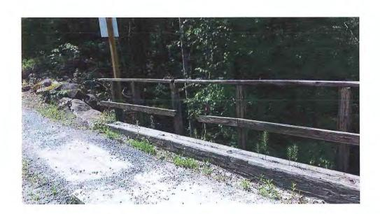
Photo 4 - Railing broken at S/W corner
