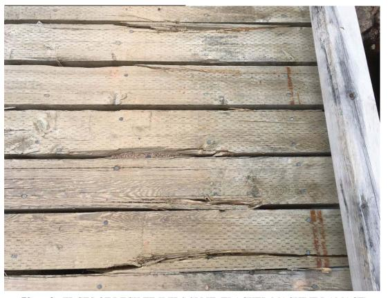
Photo 9 - EDGES OF DECK TIMBERS SPLIT (TRACKED MACHINE DAMAGE)
