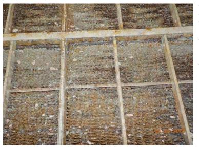
The photo to the left shows the plugging that is progressing into the "D" baskets. This will continue to degrade the performance of the air preheater rotor due to its inability to absorb flow through the sheets.
