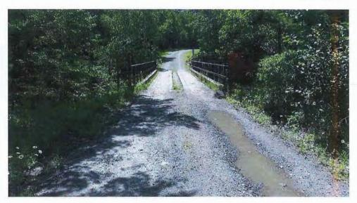
Photo I - North Approach Looking South - Rut and Edge Erosion
