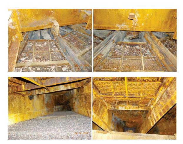
The cold end grating that supports the cold baskets appeared in good condition. The grating sits on blocks that are welded to the diaphragms. The grating free floats on these blocks so that it does not restrict expansion of the rotor under load.
