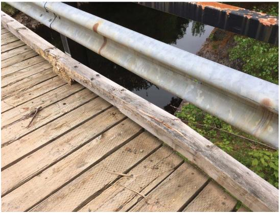
**Photo 8** - BROKEN WHEEL GUARD SW CORNER
