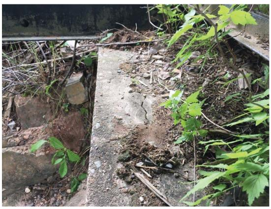
**Photo 16** - LONGITUDINGAL CRACK ON TOP OF E ABUTMENT Date Filed: November 29, 2018 Page 246 of 1289 REDACTED
