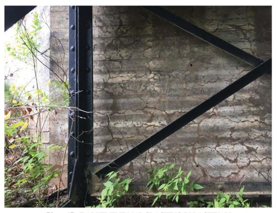
Photo 17 - E ABUTMENT MAP CRACKING IN BACKWALL
