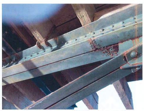
Photo 13 - APPARENT REPAIR TO BOT FLANGE OF TOP CHORD, E SPAN
