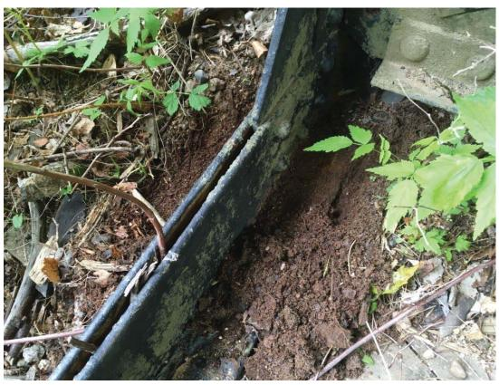
Photo 10 - TRUSS BEARINGS BURRIED IN DEBRIS AT E ABUTMENT Date Filed: November 29, 2018 Page 243 of 1289 REDACTED
