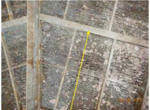
These strips are covering gaps that persist around the basket perimeter and are a stop gap measure for pressure loss and loss of return. They also cover the ends of the stay plates and prevent weld inspections. No issues were found at these locations, but the problems persist because the baskets are small for the compartments.
