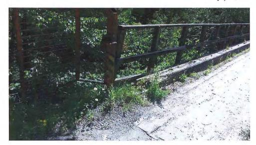
Photo 7 - Wheel Guard and railing broken at N/E corner
