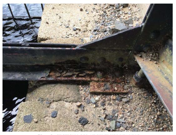
Photo 9 - SECTION LOSS AT SW TRUSS BEARING
