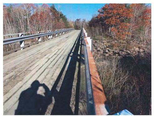
Photo 3 - MINOR BEND IN SE BRIDGE RAIL
