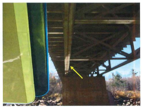
Photo 9 - LOOKING AT MINOR BEND IN E BOT CHORD OF N TRUSS
