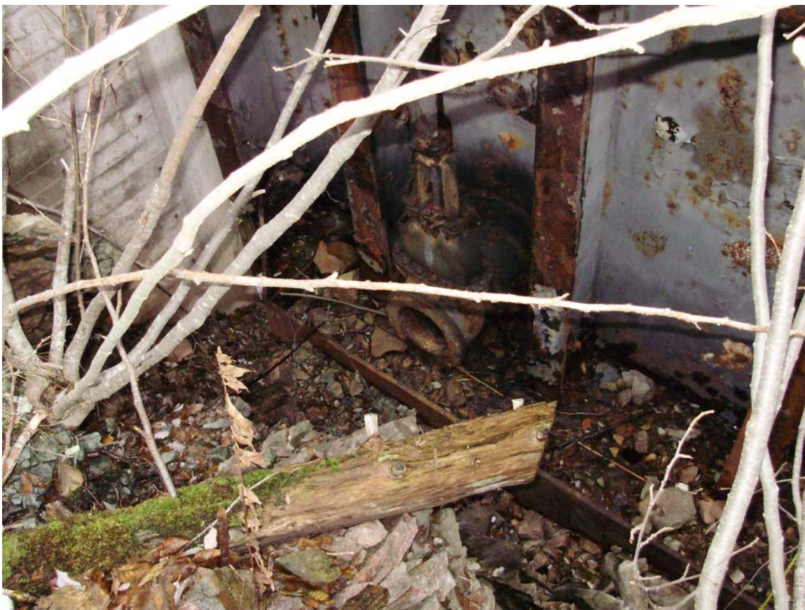
Photo 18: Downstream face of gate with gate valve used for filling the tunnel
