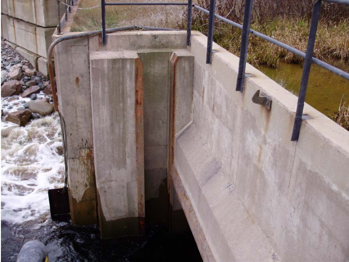
Photo 1: Gate gains and soffit on right side
