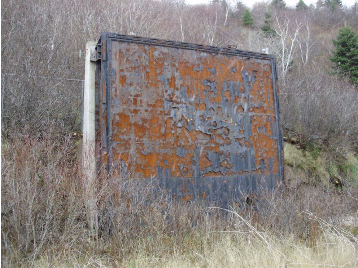
Photo 6: Overview of tailrace gate located adjacent to the tailrace tunnel portal. Upstream face of tailrace gate shown here.
