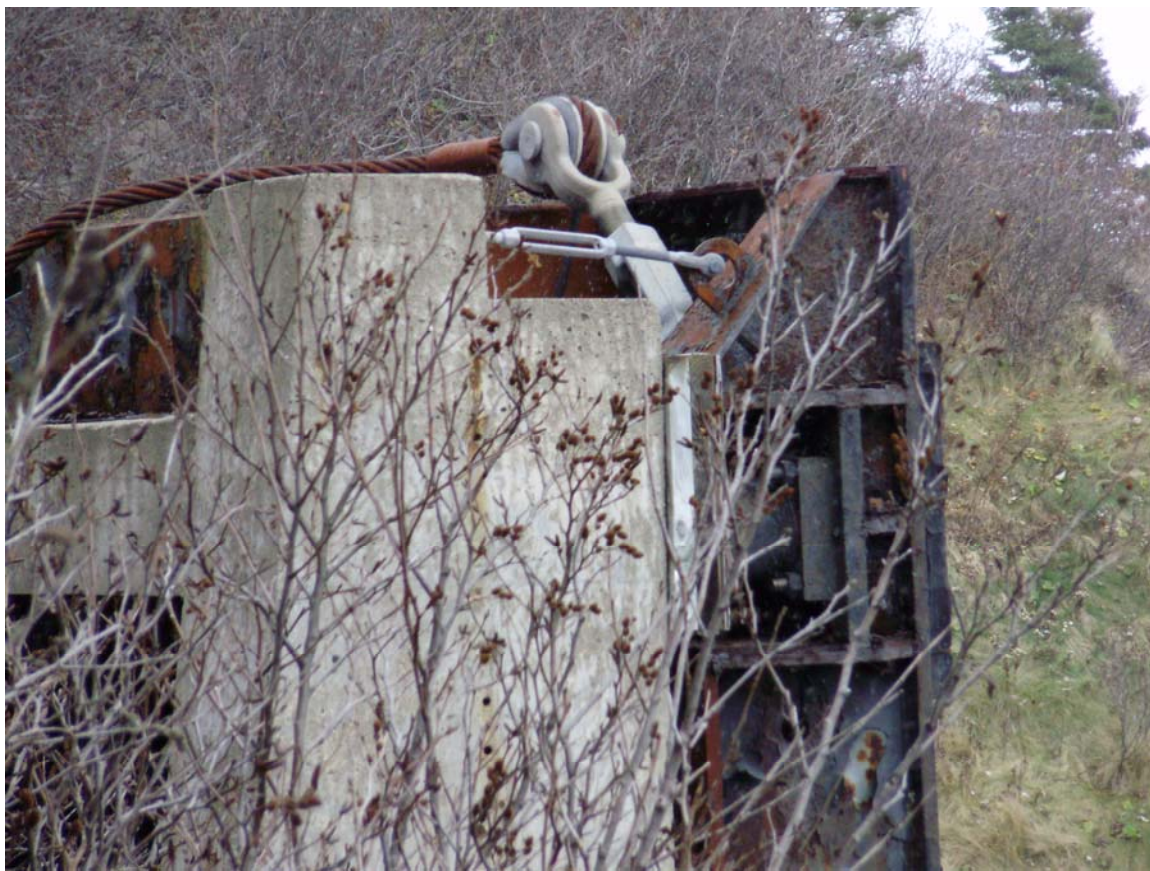
Photo 24: Turnbuckle at upper left corner of gate
