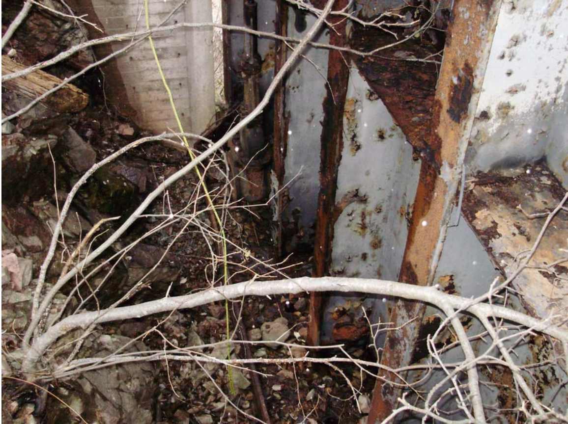
Photo 19: Downstream face of gate, right side, showing rock and debris accumulation on bottom horizontal member. Debris is more than 2 ft deep.
