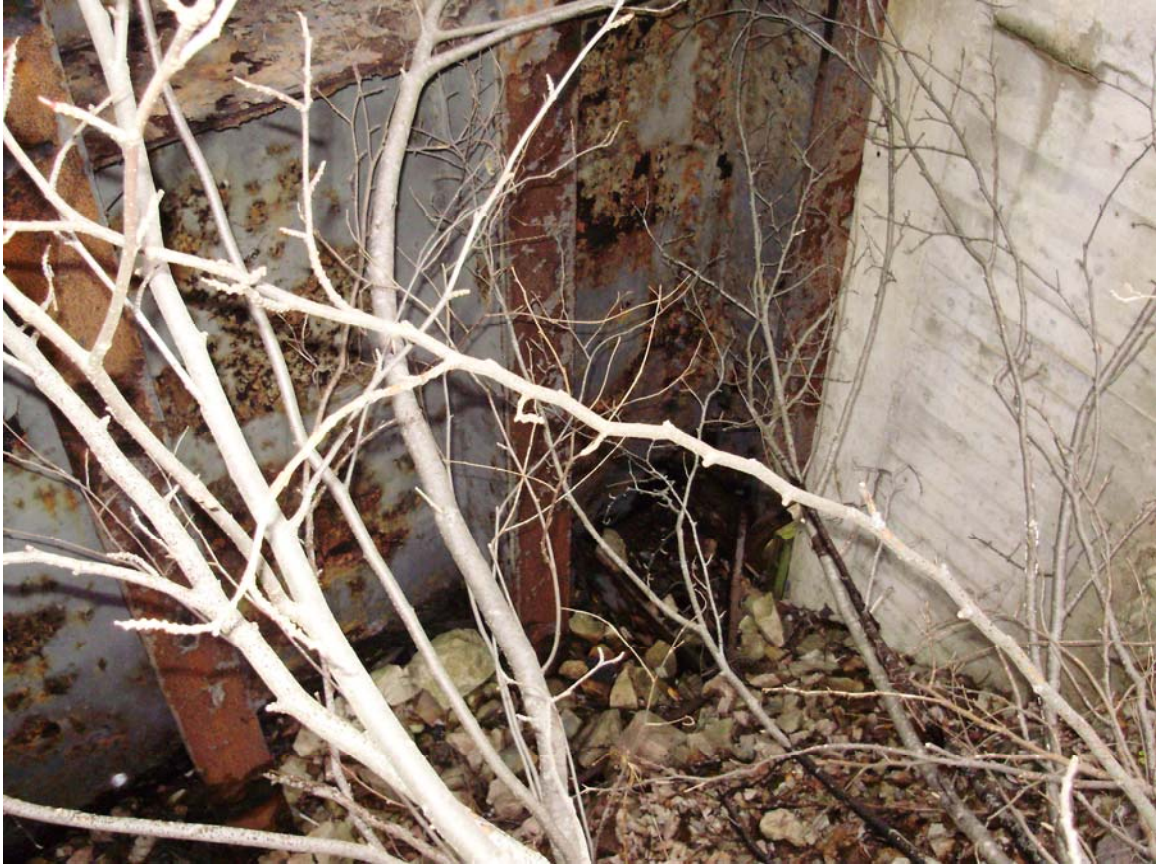
Photo 20: Downstream face of gate, left side, showing rock and debris accumulation on bottom horizontal member. Debris is more than 2 ft deep.
