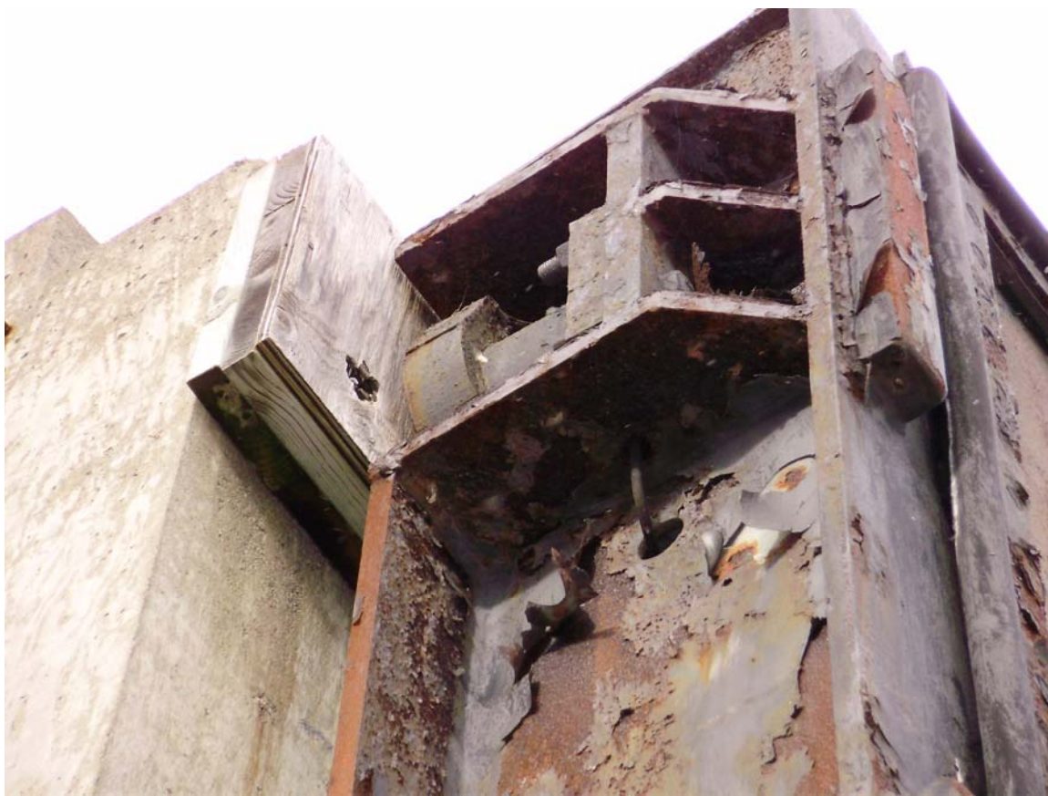
Photo 16: Upper left hydraulic cylinder
