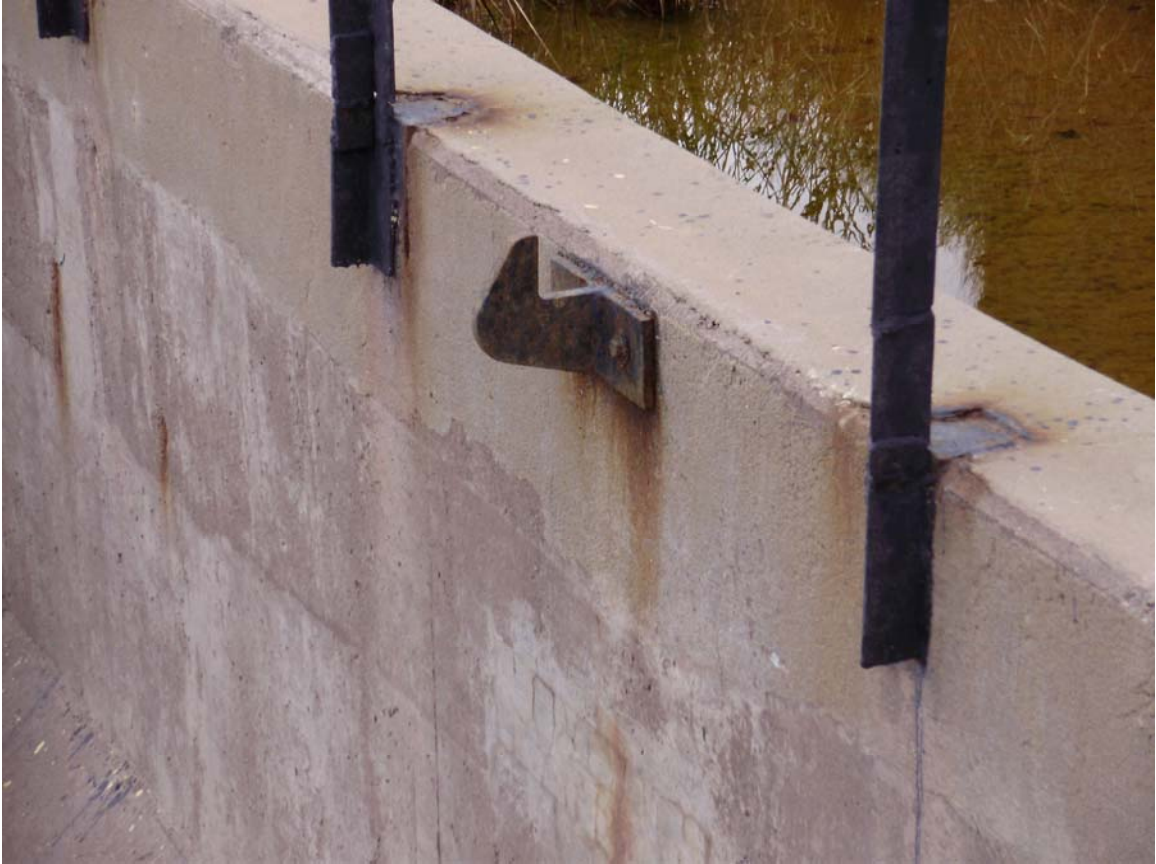
Photo 4: Support for gate sling when gate is in position
