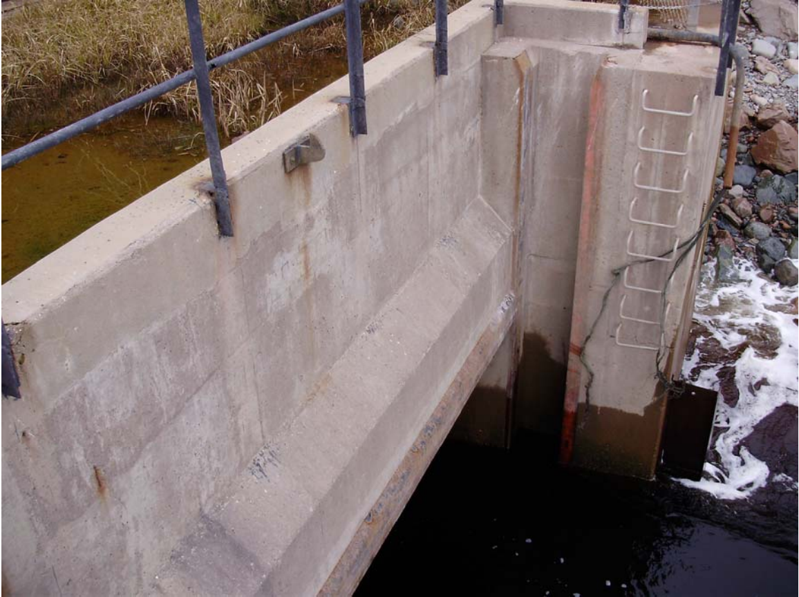
Photo 2: Gate gains and soffit on left side
