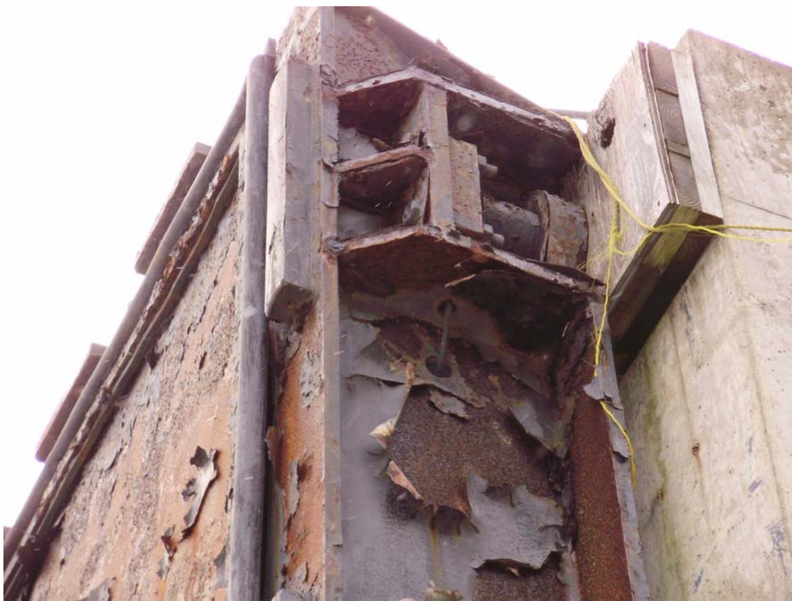
Photo 13: Upper right hydraulic cylinder. Note the hydraulic line below the cylinder.
