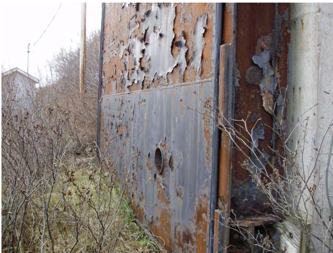
Photo 9: Upstream face of tailrace gate – lower half
