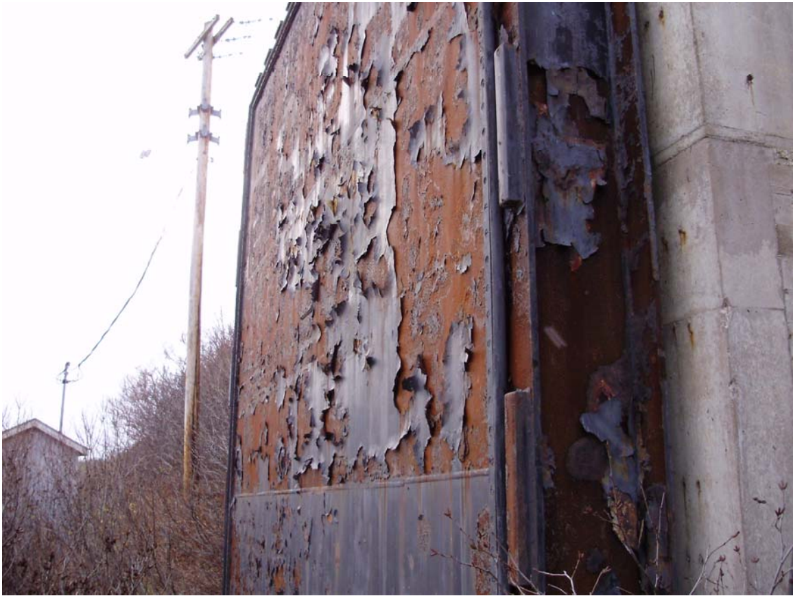
Photo 8: Upstream face of tailrace gate – upper half
