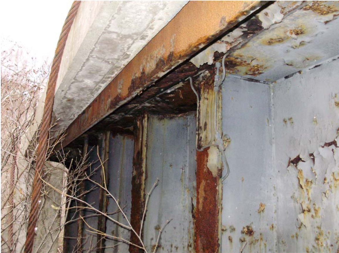
Photo 21: Downstream face of gate showing top horizontal structural member, hydraulic lines and lifting sling
