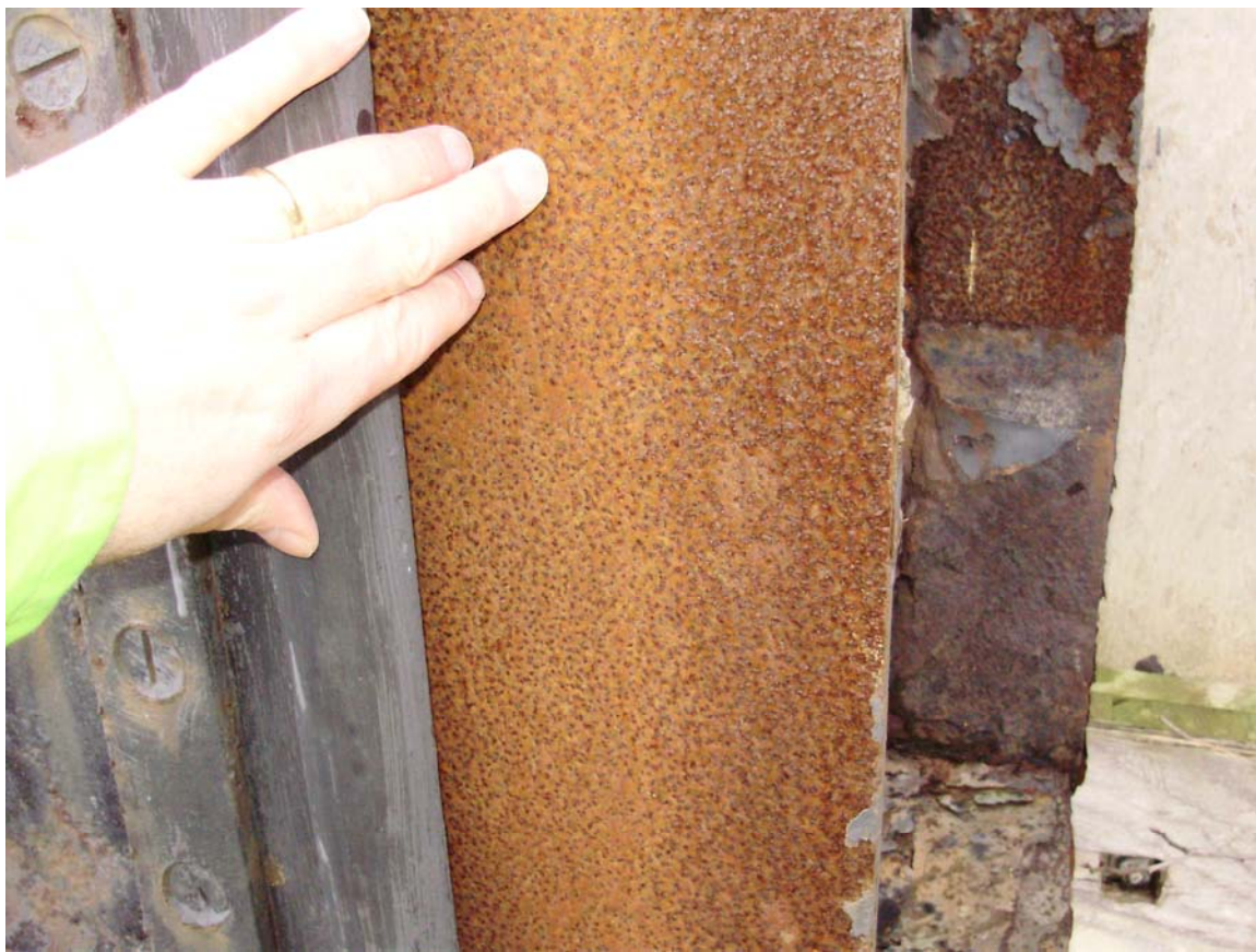
Photo 11: Close up of right side of tailrace gate showing bare metal and the starting of pit corrosion.
